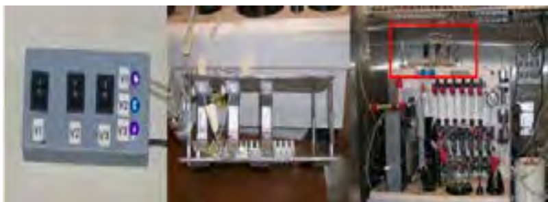
Photo 1. Three electronic three-way valve V1', V2' and V3'
